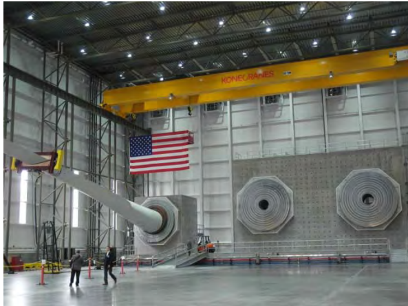
Large Blade Facility, Boston, MA
